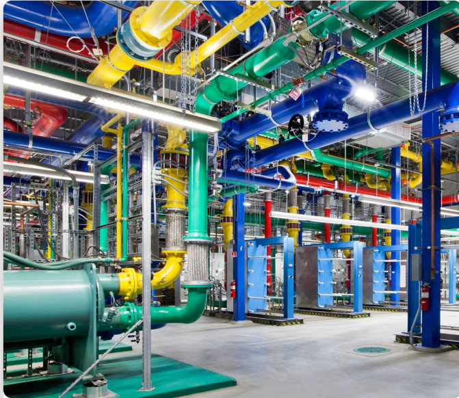
Cooling system of a data center Google, Oregon, 103 MW
