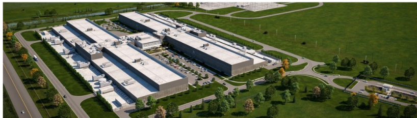
Figure 1: Depiction of Meta's data center in DeKalb, IL, USA where low-carbon concrete discovered by artificial intelligence methods has been tested.
